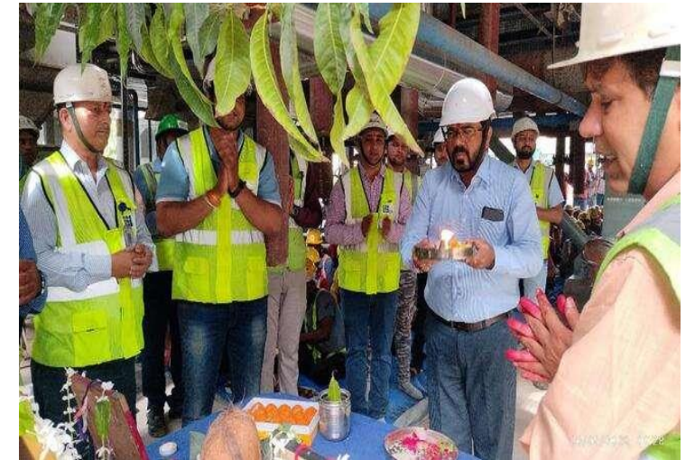
Boiler-1 Light up Pooja Ceremony
